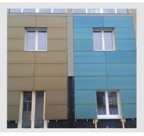
With Kromatix<sup>TM</sup> technology, the solar panels are no longer architectural intruders. They can be harmoniously integrated into the building envelope. Roofs, facades and balconies are now fully available to collect the sun radiation and maximize the solar energy production.
